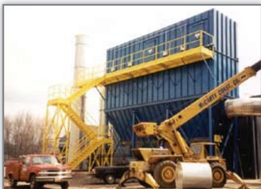
960 Bag Pulse Jet Collector with 15,700 Ft 2 of Cloth Mold Fume Line - High Density Polyester at 110°F
